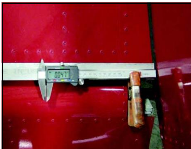
Figure 7.1: Inspect Rear Spar Doubler
